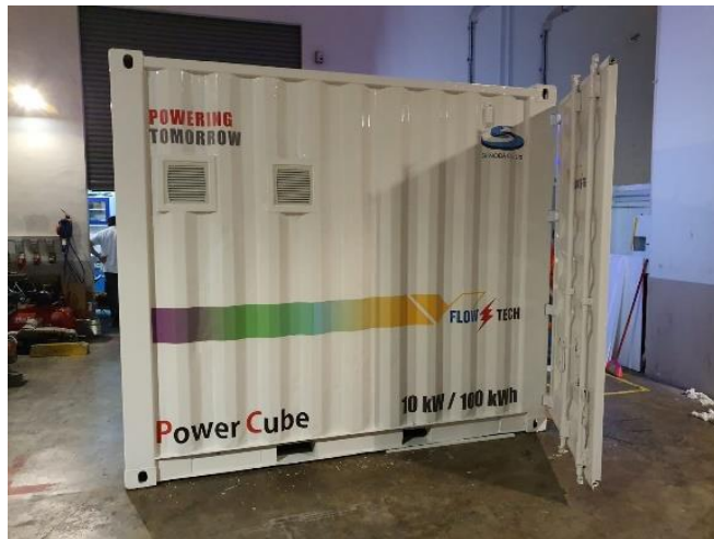
Caption: A 100kWh Vanadium Redox Flow Battery ESS
