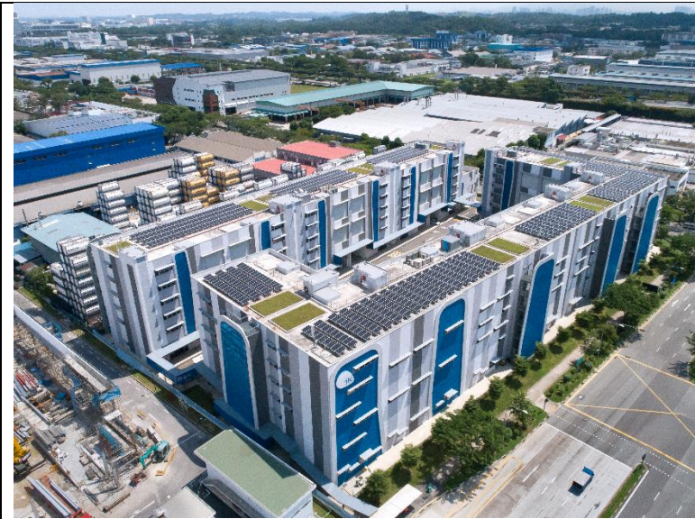
Aerial view of the SolarRoof installation on JTC Space @ Gul.
