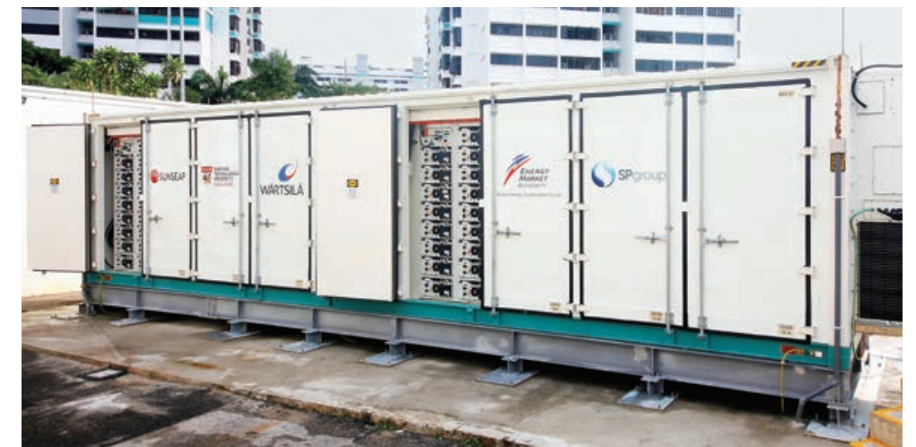
^ The utility-scale ESS test-bed funded by EMA and SP Group will evaluate the performance and safety of ESS in Singapore’s hot and humid environment.
