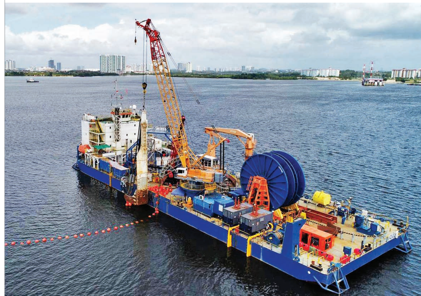
^ Laying of subsea cables interconnecting Singapore and Malaysia.
