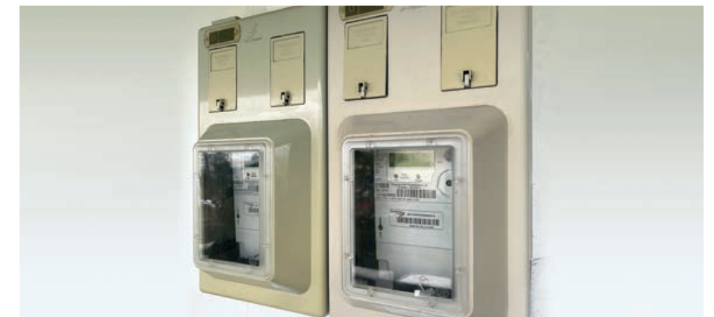
^ By 2024, all households in Singapore will be installed with advanced electricity meters to track their half-hourly electricity usage.
