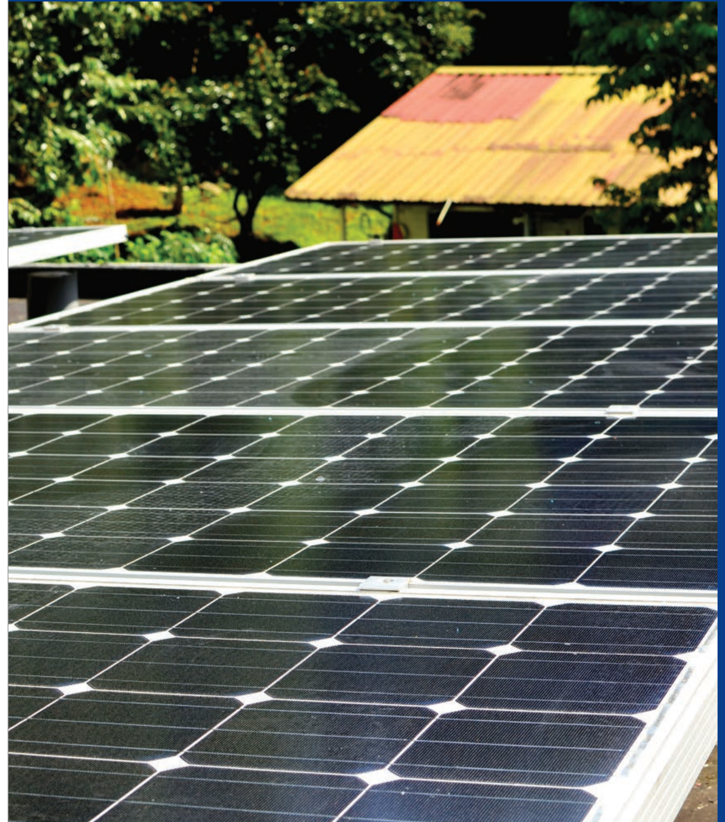
^ EMA is working with the industry and research community to understand the potential of micro-grids, such as assessing the reliability of electricity supply within a micro-grid infrastructure using solar photovoltaic technology with the Pulau Ubin micro-grid test-bed.
