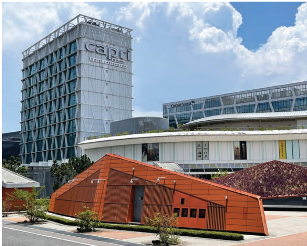
^ The 66kV Changi Business Park substation delivers electricity to consumers in the area.
